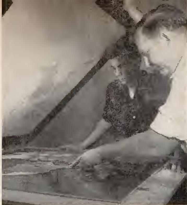
Geographer's layout of a hemisphere is transferred to flat sheet of plastic by a silk-screen process
